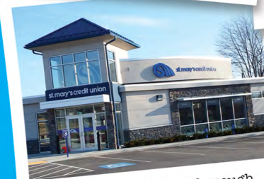
96 Turnpike Rd, Westborough
